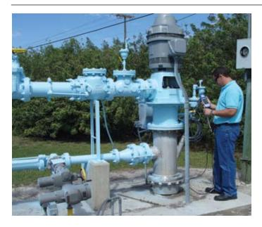
Lee County Utilities (LCU) in southwest Florida is pioneering an ambitious Aquifer Storage and Recovery program. LCU will use self-powered Aqua TROLL® 200 Instruments to monitor and communicate well level and specific conductivity measurements by SCADA or cellular telemetry. A RuggedReader® Handheld PC with Win-Situ® Mobile Software allows operators to review and evaluate measurements onsite.
