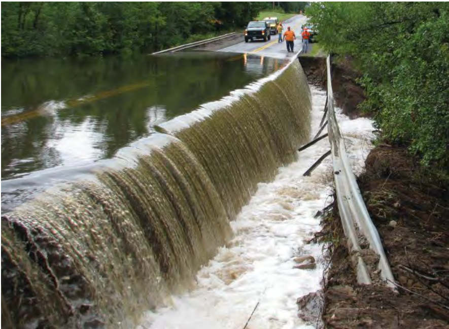
2010's late-summer flood took out not only beaver dams upstream, but also part of CR 47. The aging culvert beneath the road could not handle all the water.
