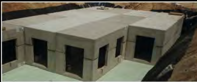
Storm Capture Detention/Infiltration
