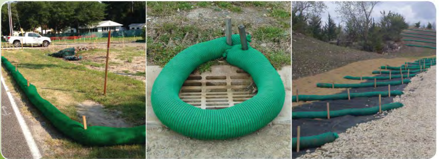
SiltSoxx ™ for perimeter control, inlets, and ditches
