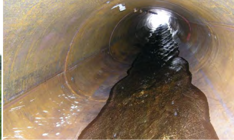
Right: The InfraSteel liner fully installed. The pipe caps on the roofline were insertion points for the flowable fill mix. Once the mix had set completely, the caps were sheared off and the holes welded.
