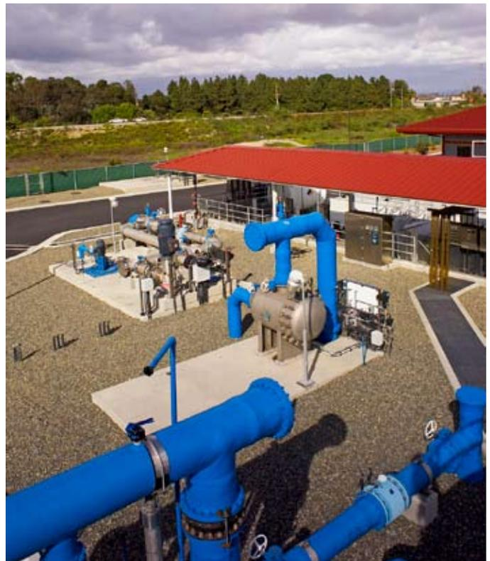
*WRD's MF/RO/UV Recycled Water Treatment Plant for Saltwater Barrier Well Injection*
