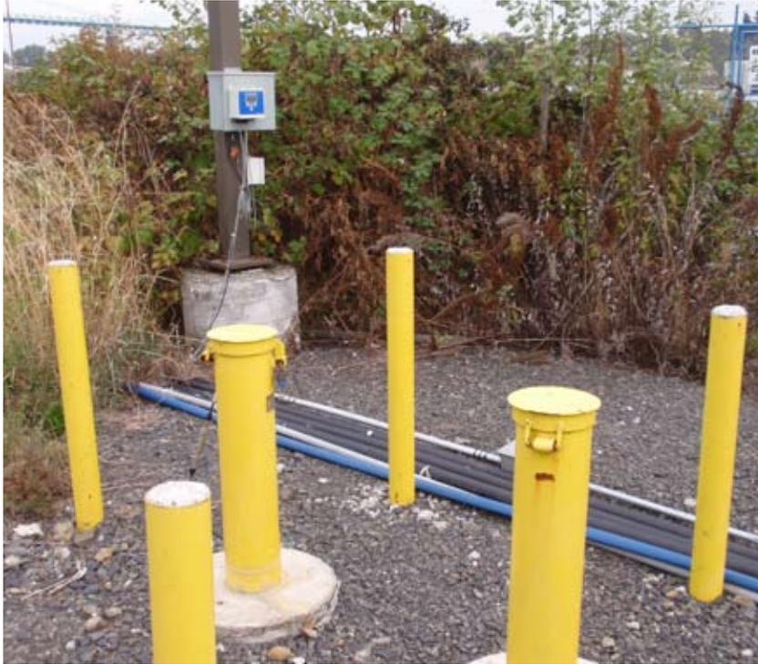
Each pumping well is equipped with a pump that is controlled by a VFD and a Level TROLL 500 Instrument. Water level elevation data generated from pumping wells is used to monitor well efficiency over time and to trigger low-water shutdown to protect pumps when water levels fall below safe pump operation levels.
