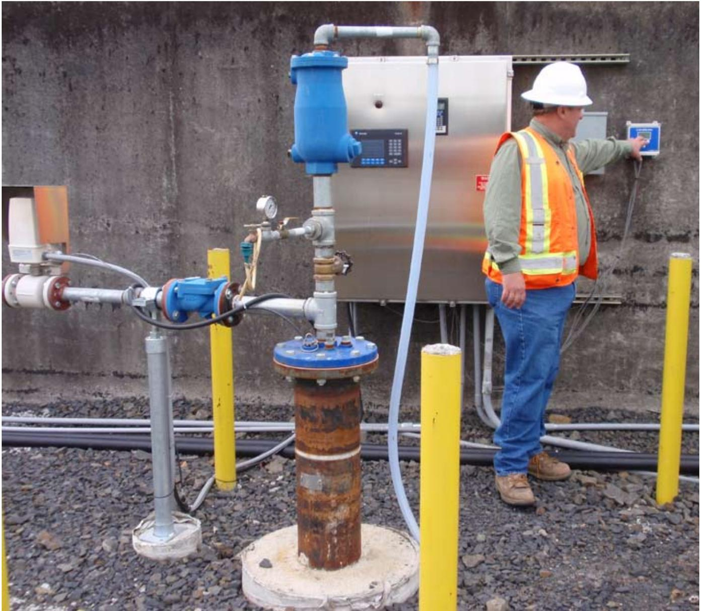
A Level TROLL 500 monitors water levels in a pumping well (foreground). The Con TROLL PRO System displays real-time water level and communicates with a PLC system. The PLC determines and directs pumping rates that will maintain the desired differential between groundwater and river elevations.
