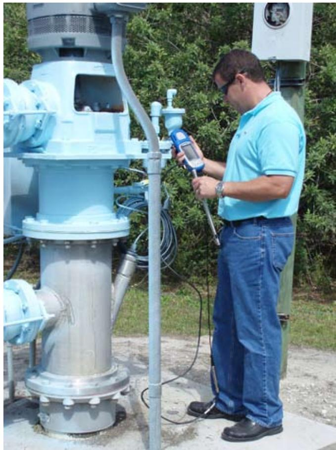
*LCU uses Aqua TROLL 200 Instruments to monitor and communicate well level and specific conductivity measurements by SCADA or cellular telemetry. A RuggedReader® Handheld PC with Win-Situ® Mobile Software allows operators to review and evaluate measurements in the field.*
